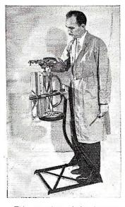
This new clamp device for lawn This new clamp device for lawn mower repairing allows the worker to have free use of both hands, by hold-ing the mower rigid in any position desired. The clamp suspends the mower at three points between the roller and tie-rod, with a snap-hoak around the center of the mower can be various positions of the mower can be changed at will without removing it from the clamp.
