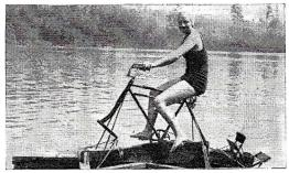
Propelled by a small paddle wheel hooked up to the pedals, this pontoon bike-boat was constructed by A. R. MacPherson.
