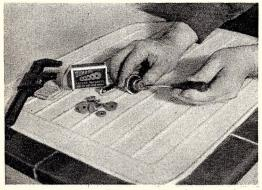
The washer is held by a single screw. Replacing it takes but a minute, and only a wrench and screw driver are necessary. An assortment of all the usual sizes of washers can be purchased for a few cents in most ten-cent stores.
